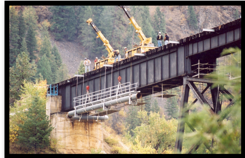
Field installation of a shop-fabricated pipe bridge
