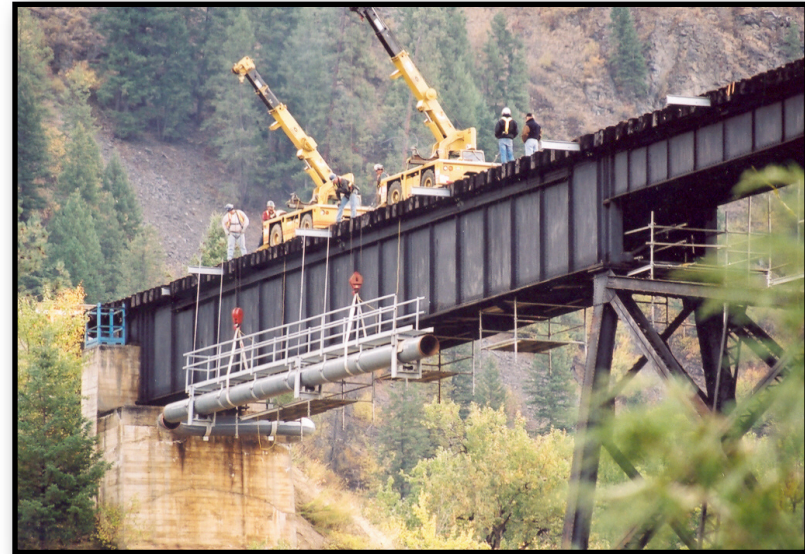
Field installation of a shop-fabricated pipe bridge
